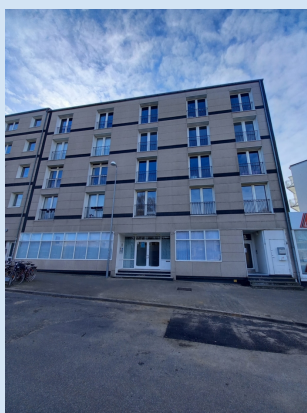
Facade mod Vesterbrogade
